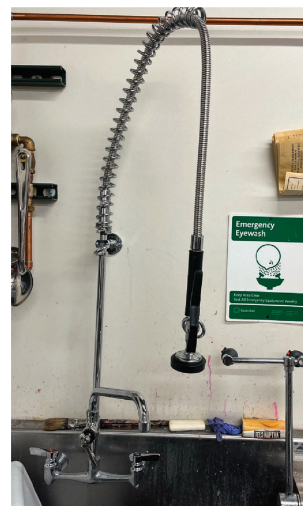
Figure 1.18 A restaurant pre-rinse sprayer and eyewash station on dye sink at Colorado State University.
